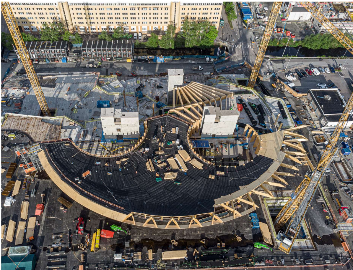
Picture 14: Birdsvie during installation of timber structure
