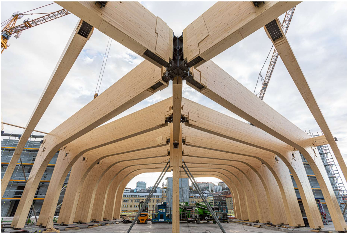
Picture 11: Cover plates around star node
