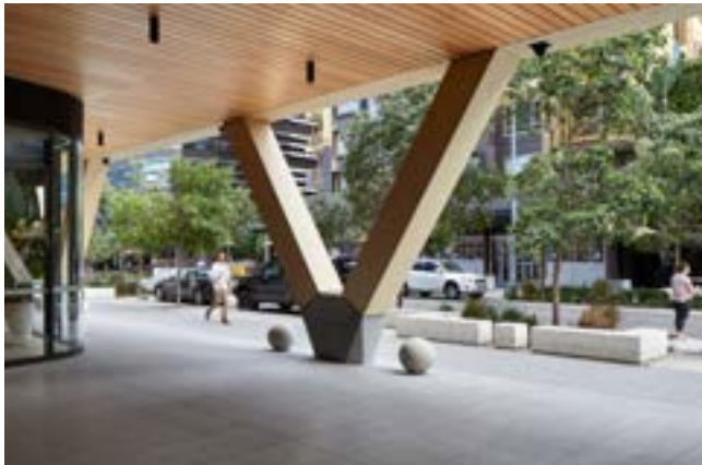
V-supports, KS Brisbane, Australia
