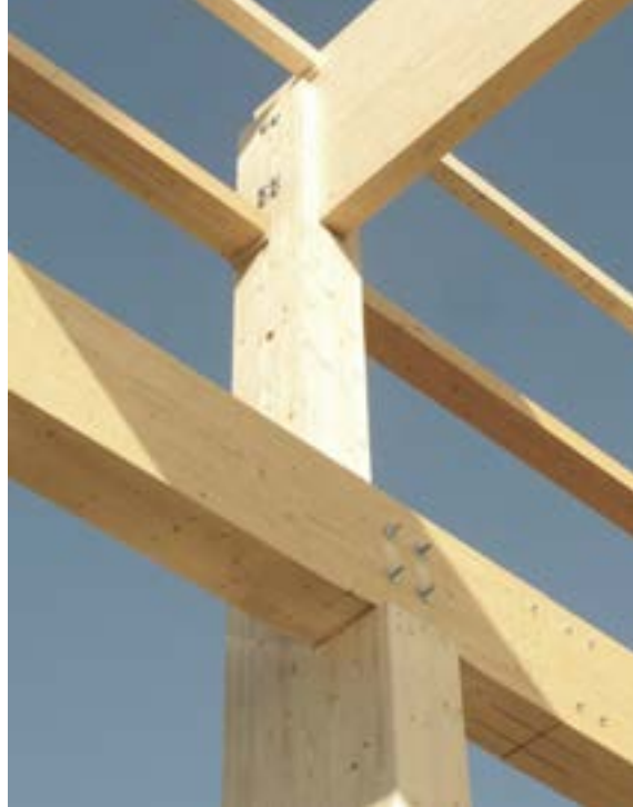
Wooden support with notch for GLT craneway. Block-bonded cross-section: 480 x 990 mm. Heavy-duty crane with loads up to 16 tonnes.
