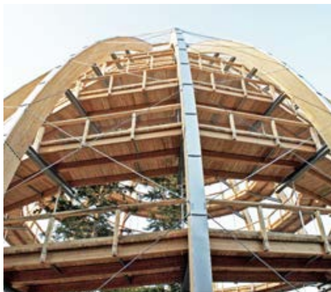
Neuschönau tree tower Curved stanchions with walkway beams
