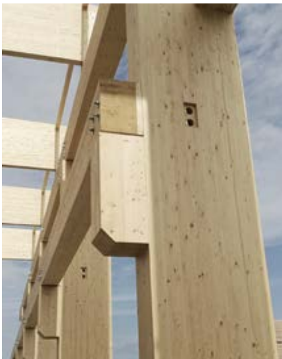
Bearing bracket in GLT design. Block-bonded craneway: 400 x 690 mm. Heavy-duty crane with loads up to 16 tonnes.
