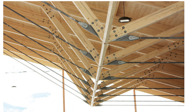
Riding school roof, Großarl Trussed parallel beams with HMR tie-bar system
