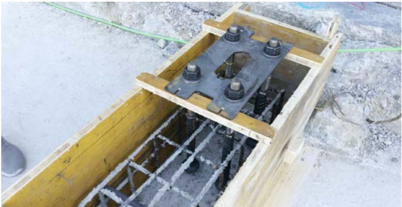
The precise alignment and arrangement of the threaded rods is achieved using a template
