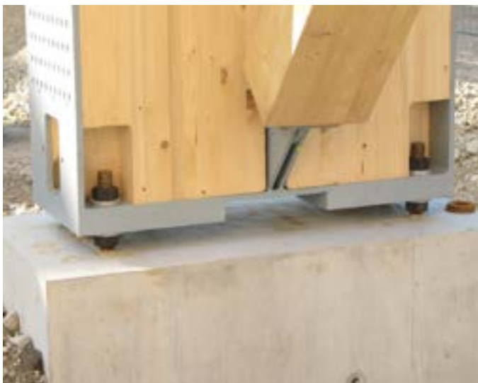
Fixed support with bracing connection
