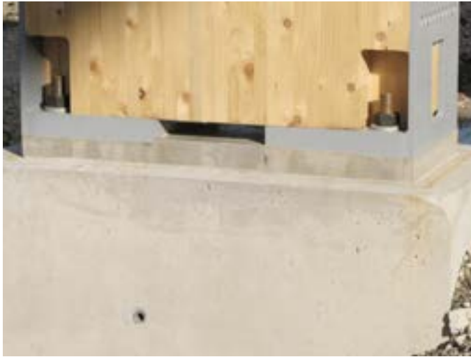
Subsequent flush fit with cast concrete
