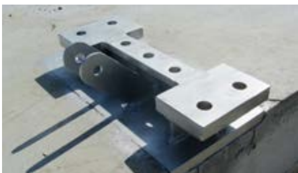
Wooden support with bonded threaded rods, welded base integrated in foundations, foot steel part calibrated and welded all round on the building site.
