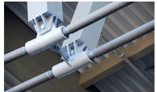
GVZ Ingolstadt rail track roofing, trussed arch beams, completely pre-assembled at factory
