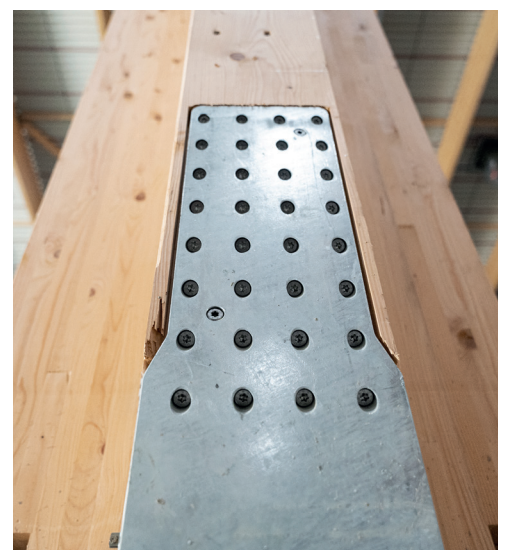
Detail of clamped timber columns
