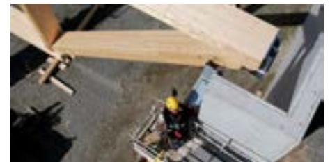
Installation of the truss by tandem lift
