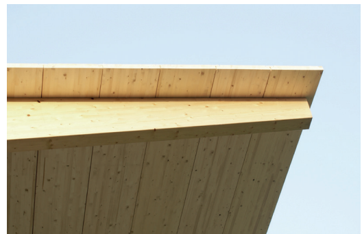
Profidec with joint strip, spruce, 600 mm covering width / 5 mm laying clearance
