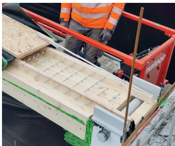
Walk-on, weatherproof covering of the compound screws possible
