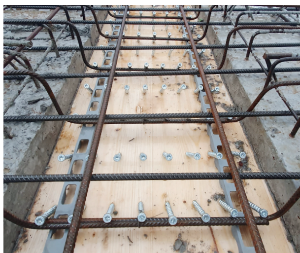
Interface between concrete reinforcement and shear
