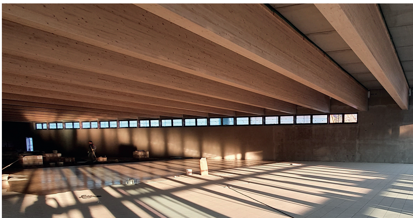
GLT structure with constructed precast ceiling
