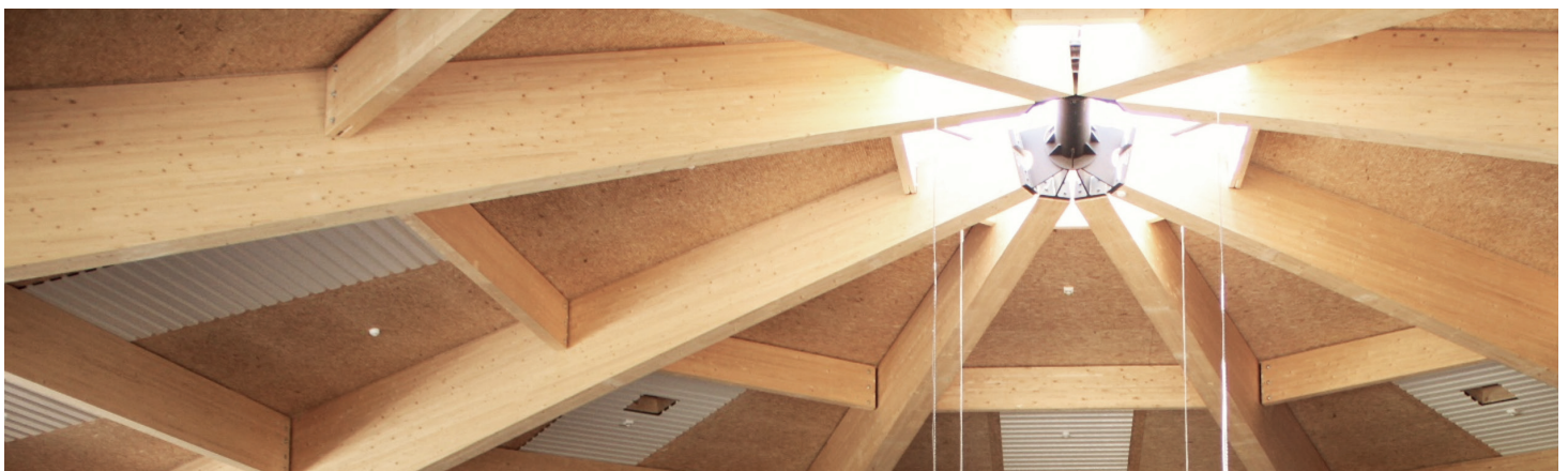
WIEHAG frame corner with central ridge hub
