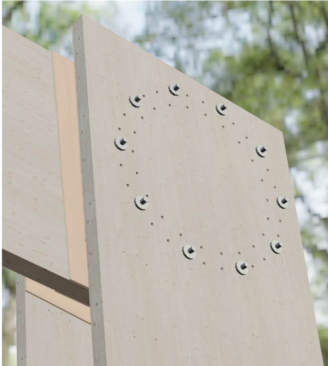
Reinforced on both sides with BFU plywood panels
