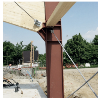
WIEHAG frame corner with steel column
