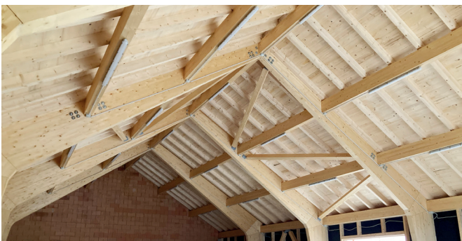
Sick Academy, Waldkirch, finger-jointed frame as roof construction
