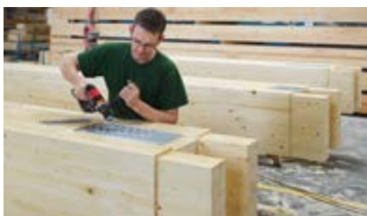
Fitting of steel parts at the factory for plug-and-play assembly
