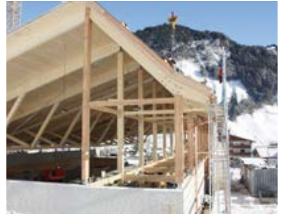
2) Spectator area with articulated columns
