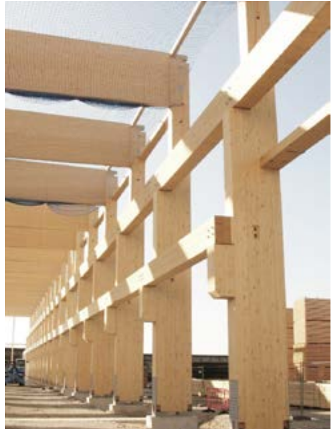
Fixed wooden supports and craneways
