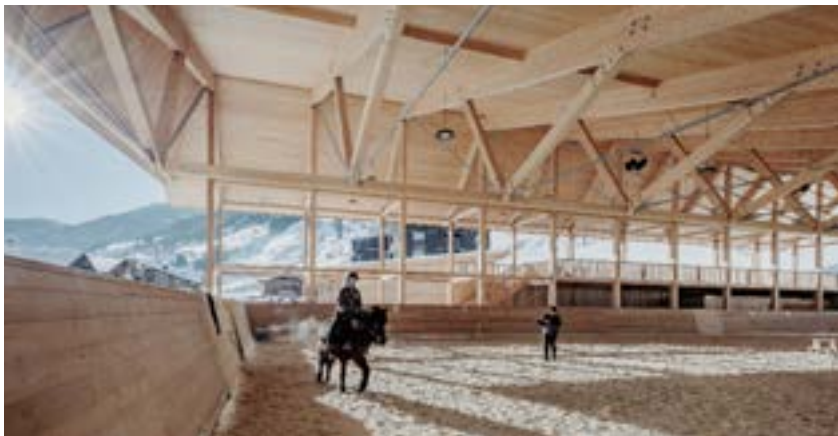
1) Gable support structure of struts and cross-laminated timber
