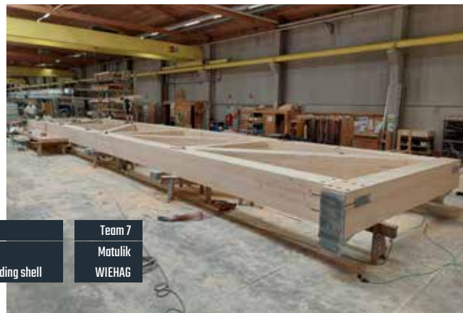
Lattice girder with a span of 25 m for the entrance area
