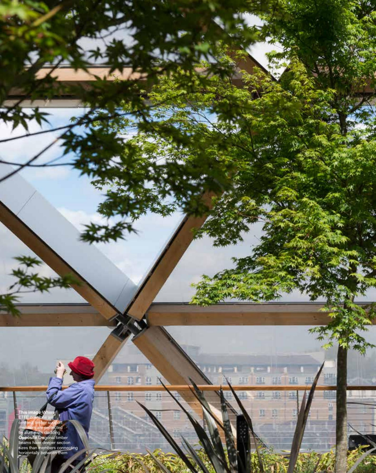
This image Where ETFE cushions are omitted, timber support members are protected by aluminium cladding
