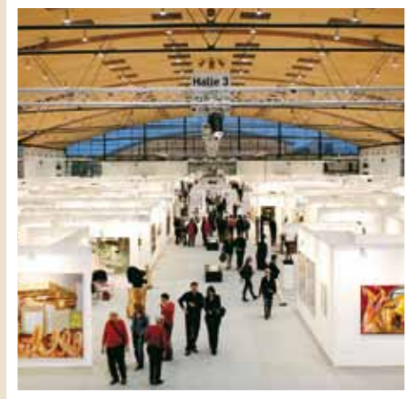
New Exhibition Hall Karlsruhe: 80 m free span arched truss, combined with WIEHAG Profiplan (as a structural, visible roof soffit)
