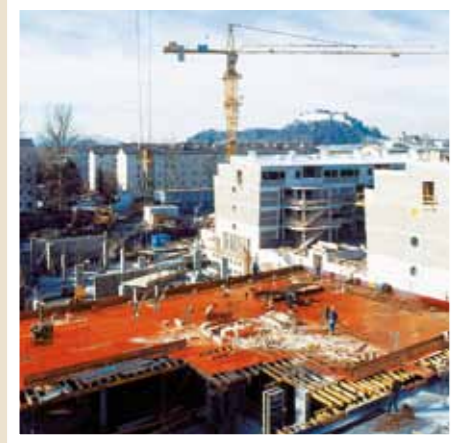
WIEHAG TOP formwork panels for a variety of custom applications (here for example in the colour red)
