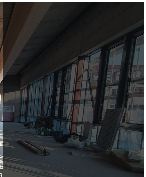
GLT structure with constructed precast ceiling
