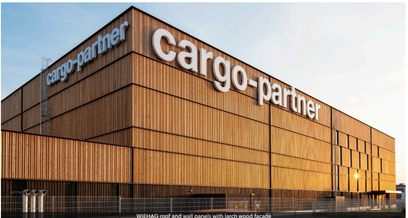
WIEHAG roof and wall panels with larch wood façade
