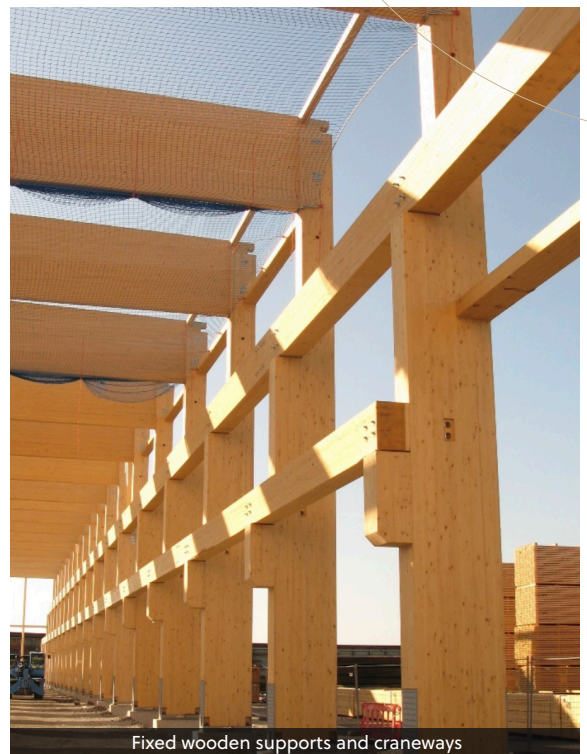
Fixed wooden supports and craneways
